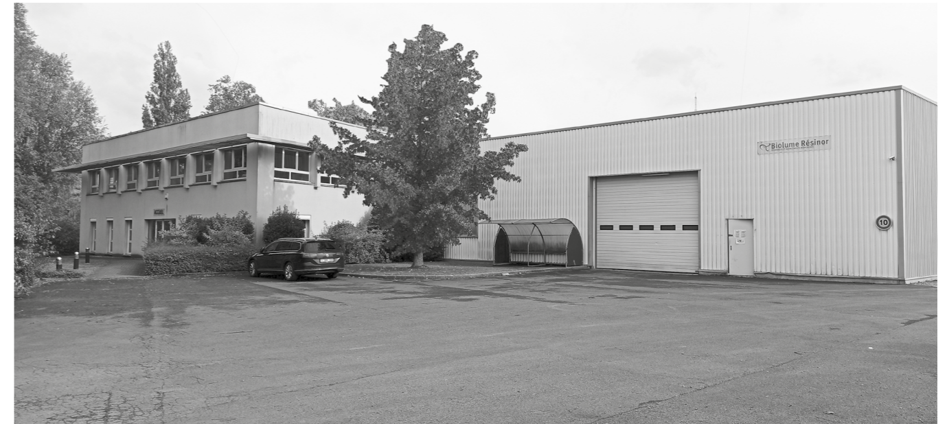
BIOLUME RESINOR, Loos site
